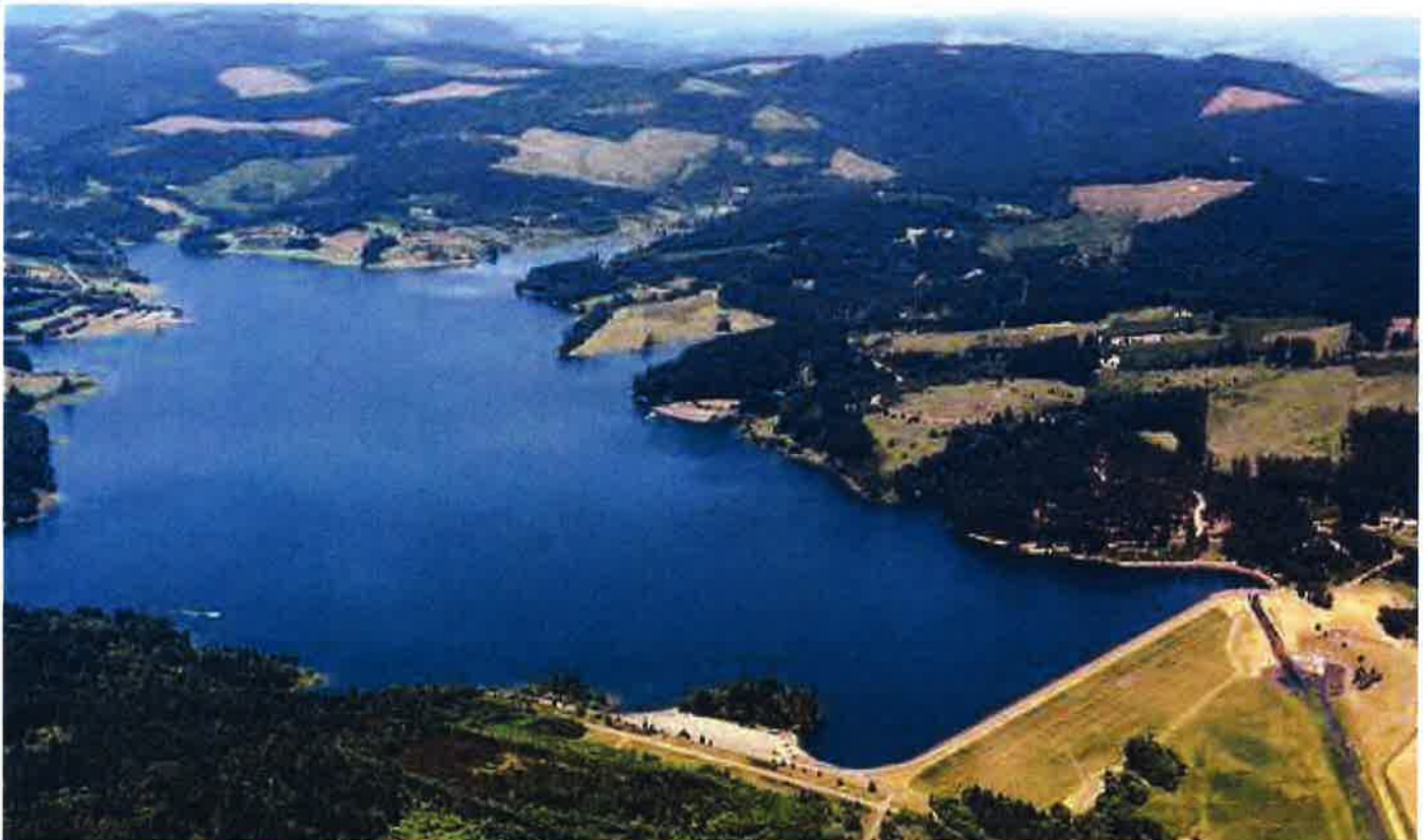
Risk Informed Decision Making (RIDM) was successfully used on the Scoggins dam project.
