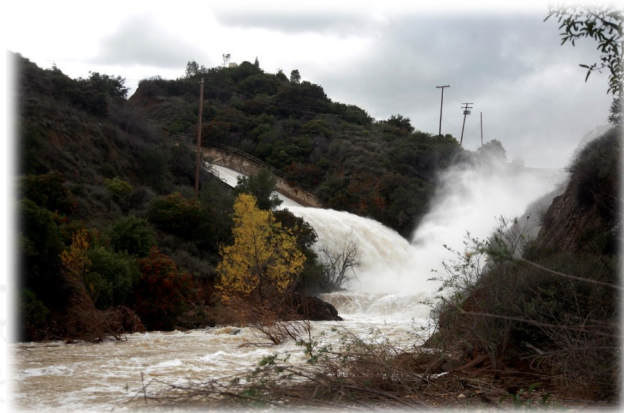
Santiago Creek Dam Spillway December 2010
