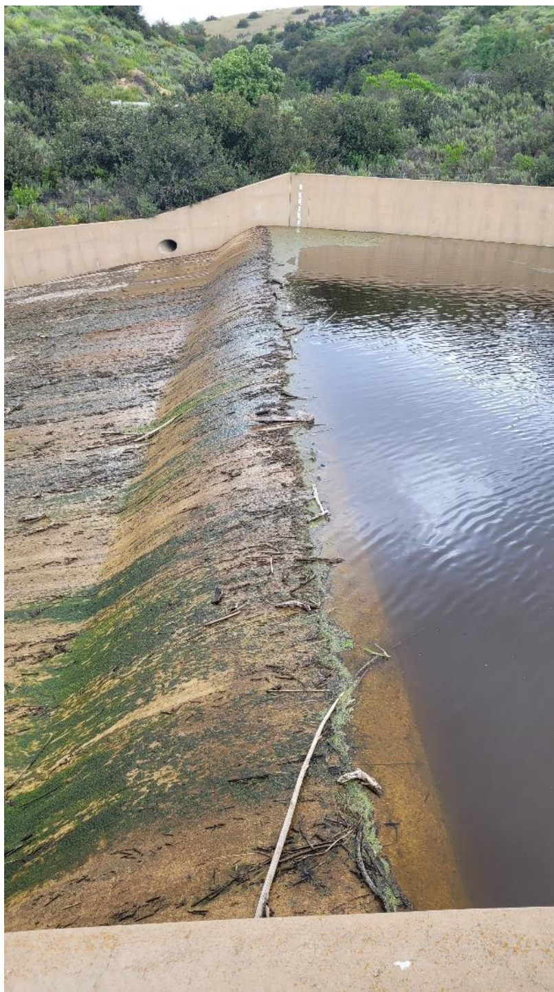
Photo 3: View of the ogee weir of the spillway.
