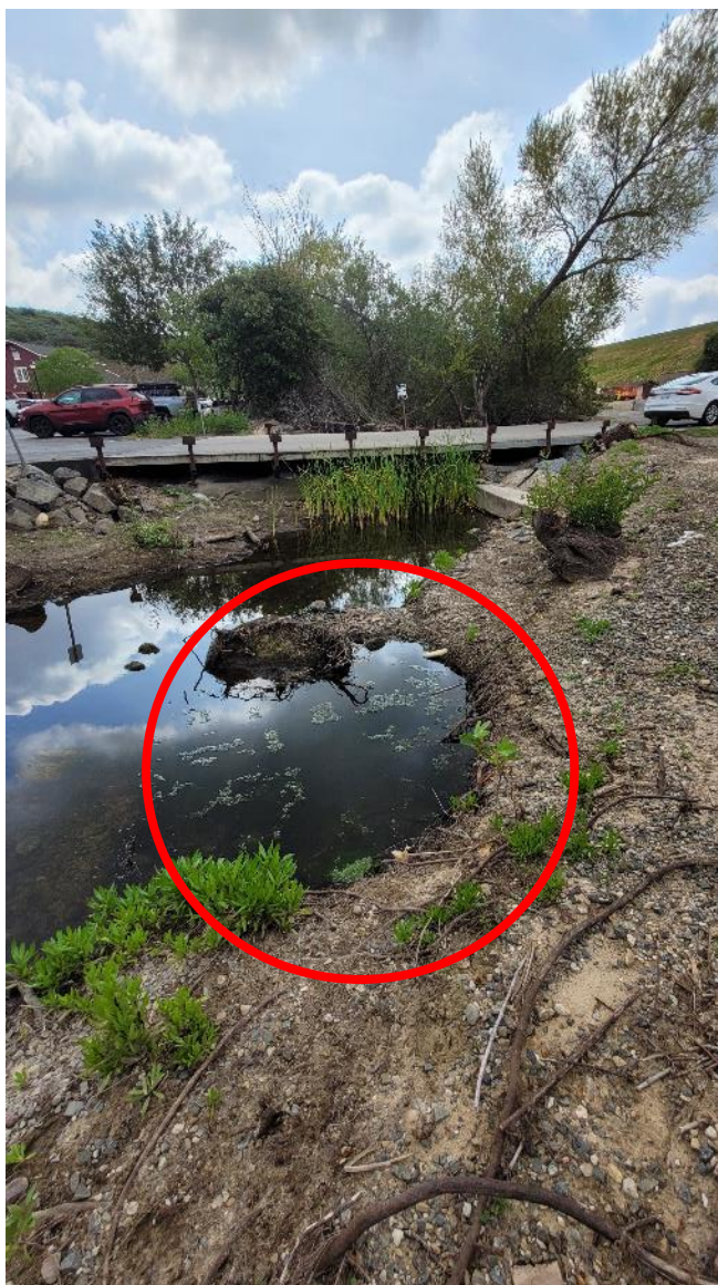
Photo 1: View of the exit portal looking upstream. The approximate location of the exit portal is circled and is underwater.
