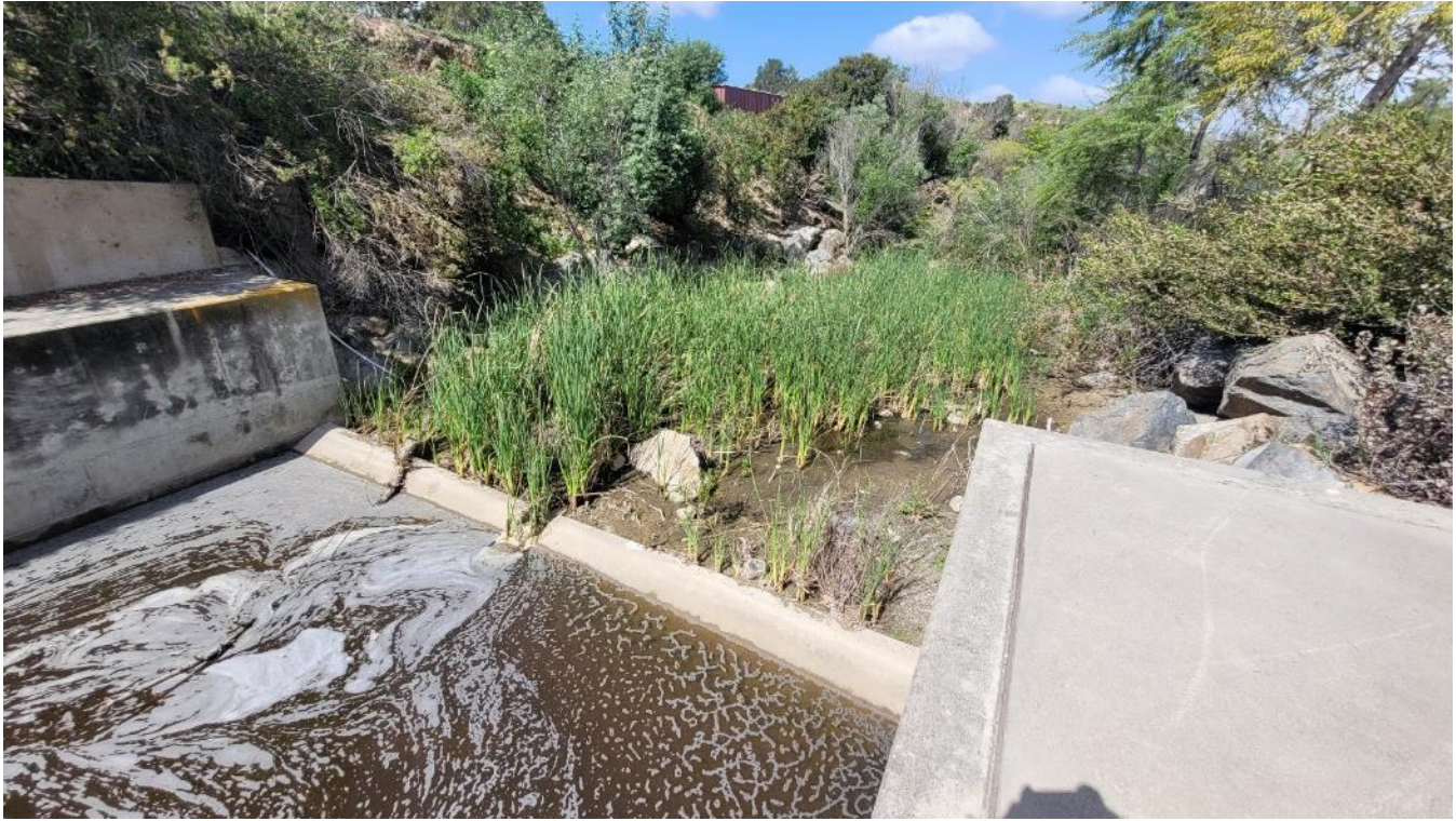
Photo 4: View of the reeds downstream of the concrete spillway channel.
