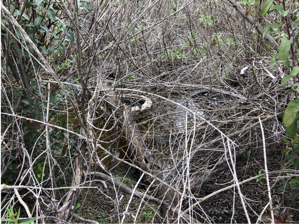
Photo 7: View of ponded area with weir near the center of the reservoir (facing west).
