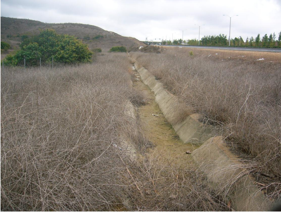
Photograph 1: Portola Drainage Channel, looking east.
