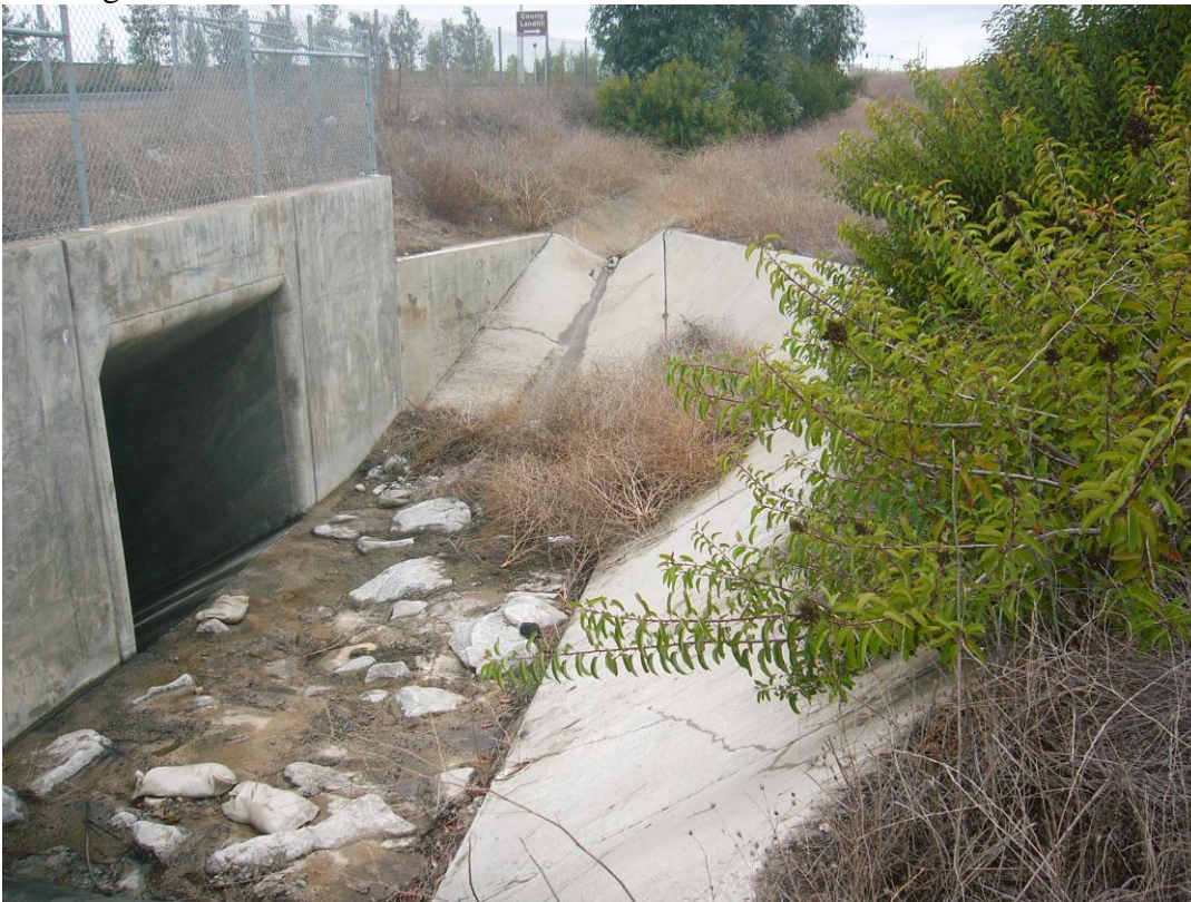
Photograph 4: Portola Drainage Channel, at Portola Parkway culvert crossing.
