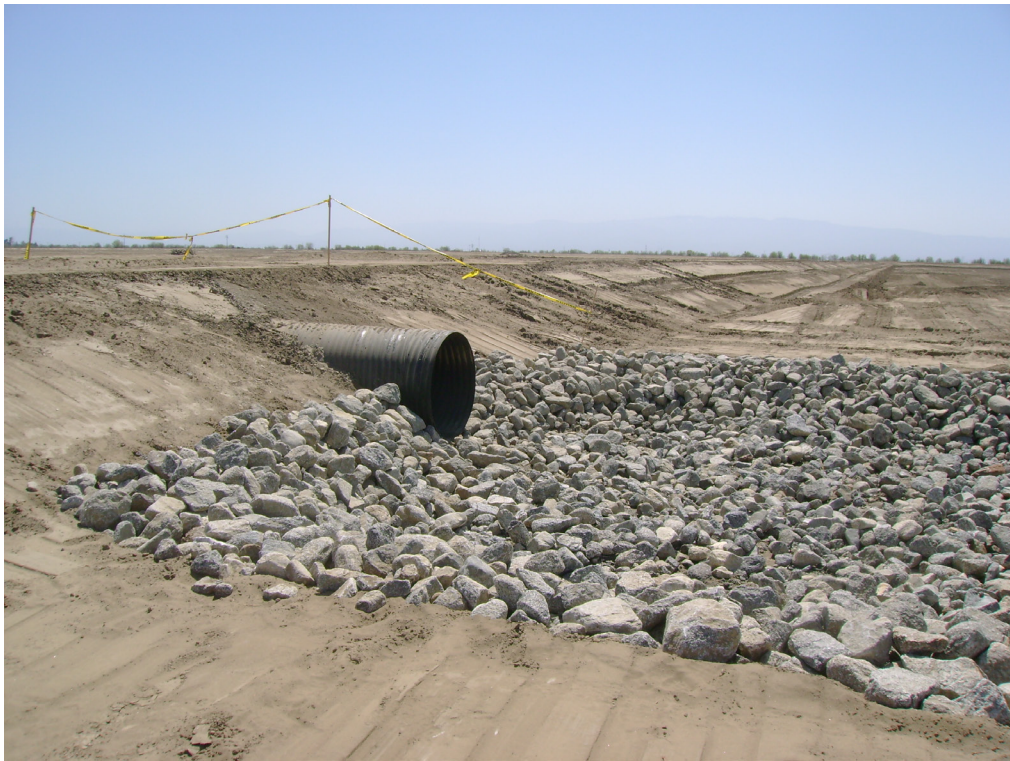
Stockdale Integrated Banking Project . 211181 Figure 2-7 Examples of Basin Transfer Structures
