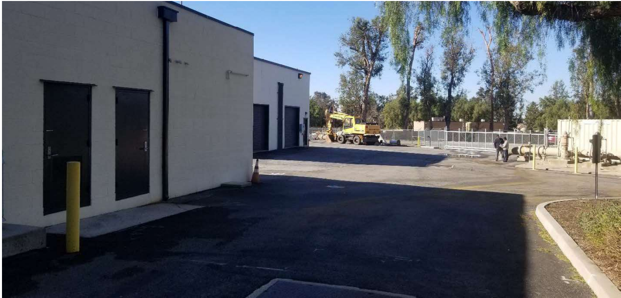
Photograph No. 2, Present site conditions within the project limit
