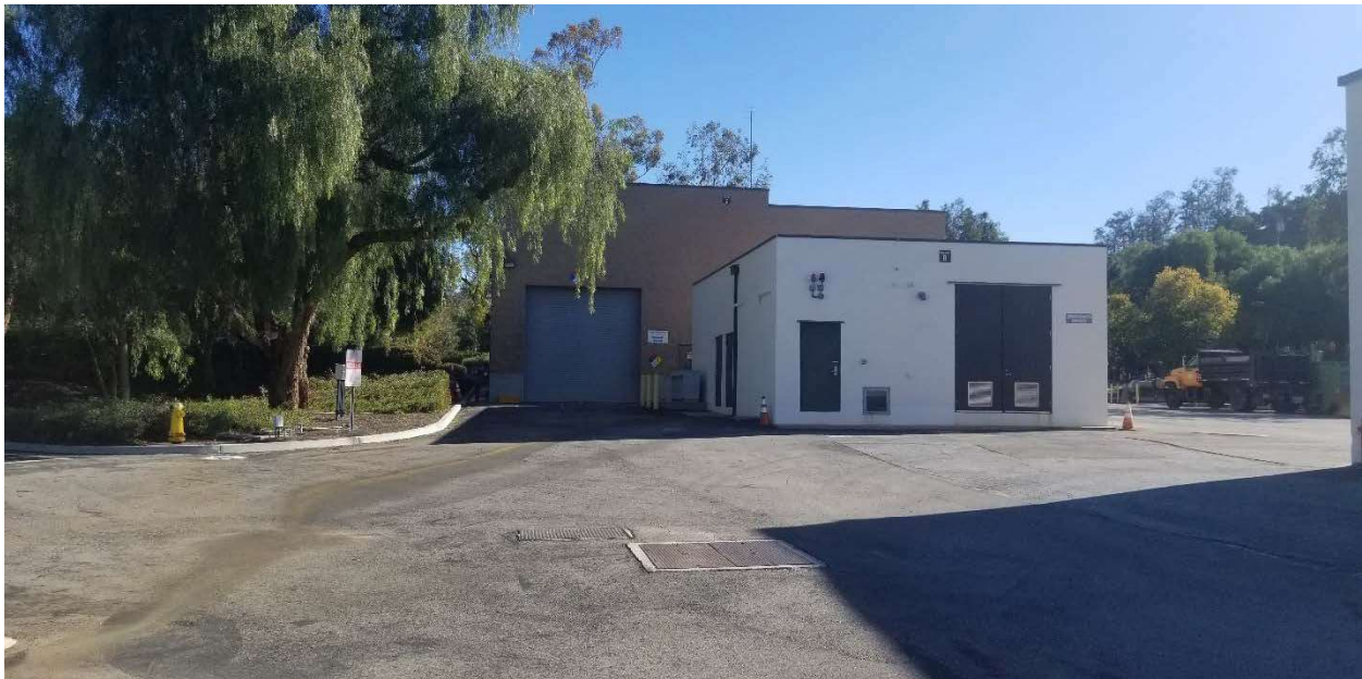
Photograph No. 1, Present site conditions within the project limit
