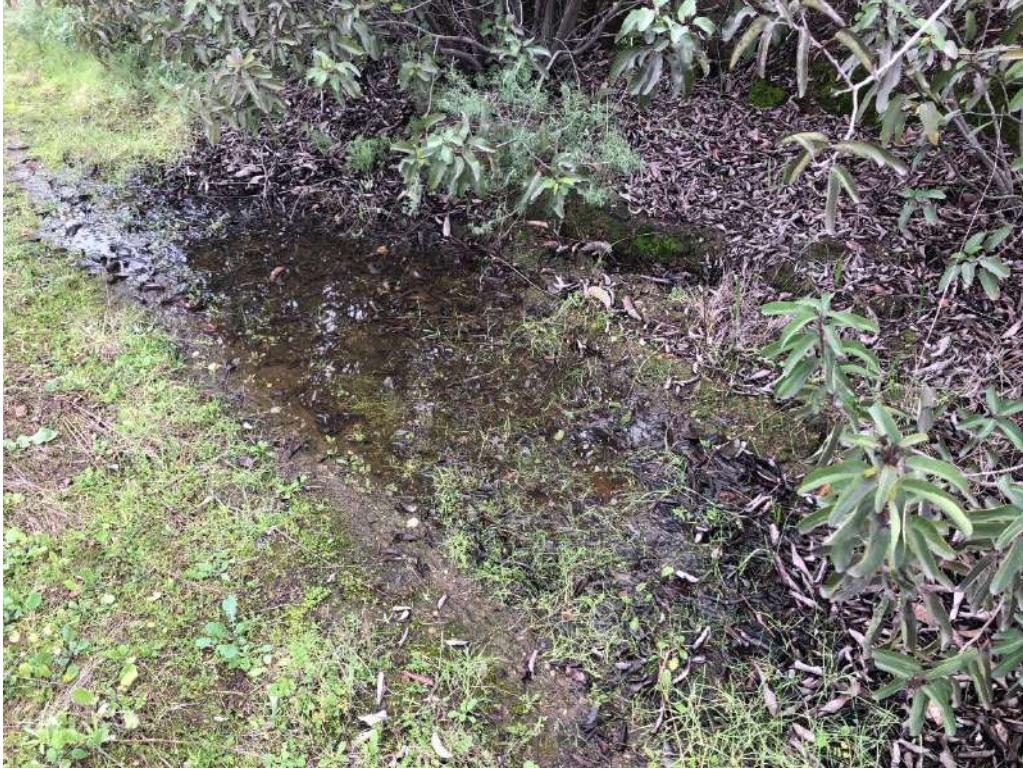
Photo 1: Puddle within the access road on east side of reservoir (facing northeast).
