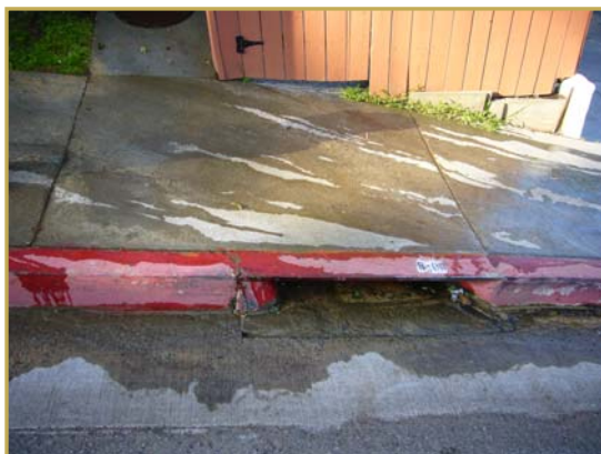
Irrigation runoff—water intended for landscape is now going down the storm drain.
