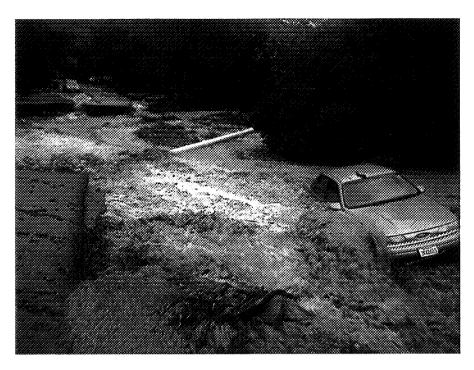
Williams Canyon (12/22/10) – Damage to Roadway and 8-inch PVC main near Creek Crossing (8-inch HDPE above-ground bypass constructed around this area)
