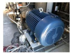
Monitor vibration records and consult the manufacturer if any excess vibration is observed.
