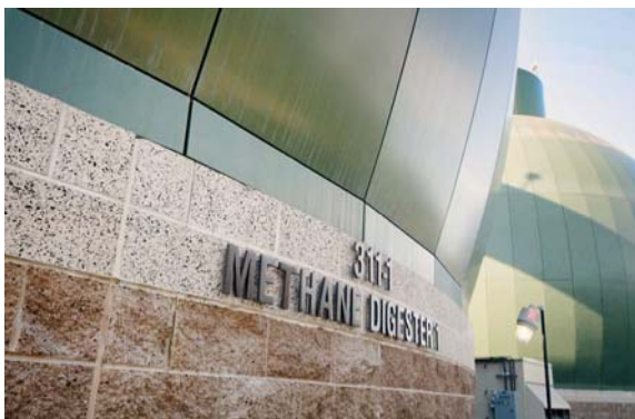
Biosolids and Energy Recovery Facilities
