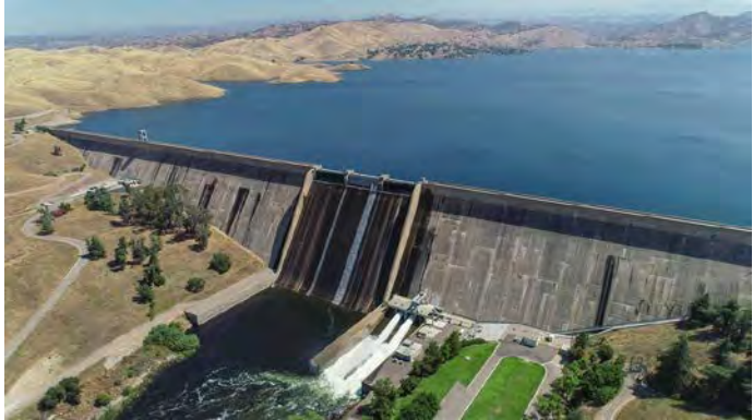
Friant Dam, Millerton Lake
