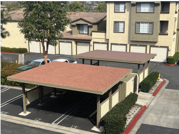
Carport Replacement • Phase 2 of 3 Complete
