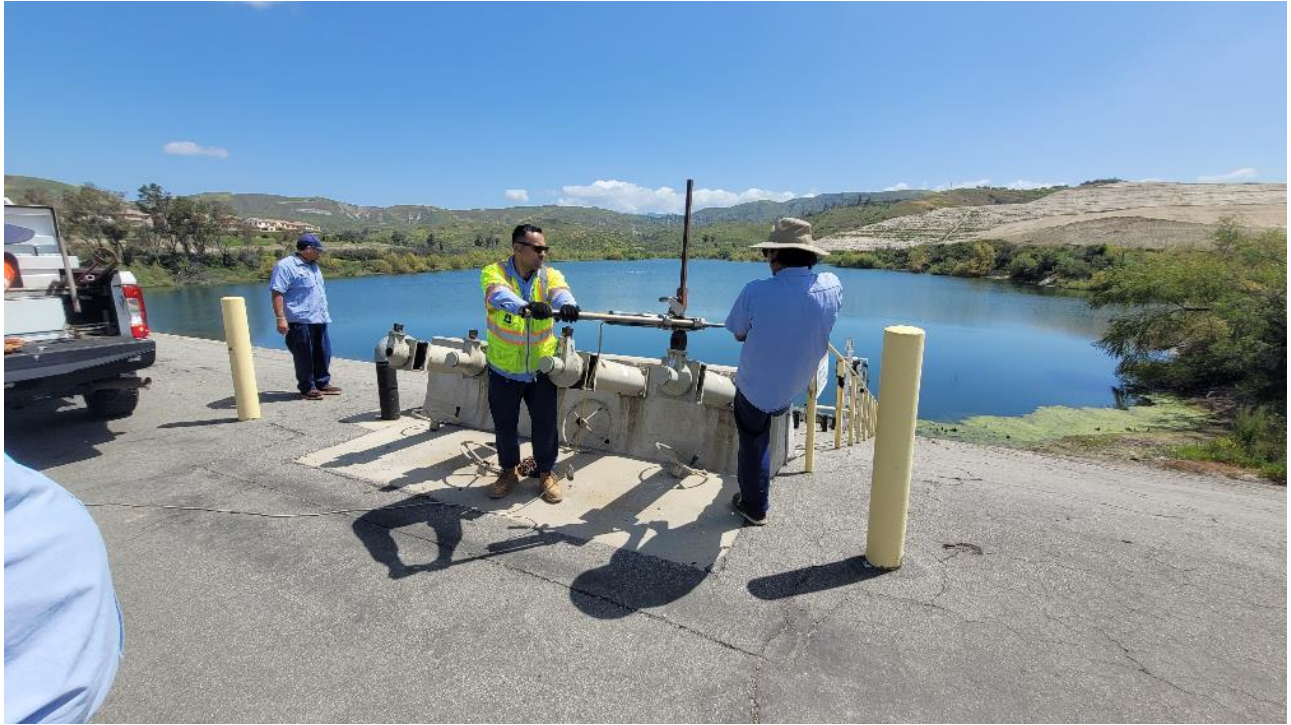
Photo 1: View of the owner cycling the upstream gates.
