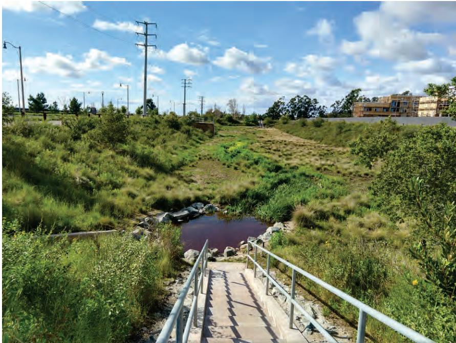
View of Parasol Park, looking west. The slopes exhibit good native diversity and cover; however, sow-thistles are prevalent throughout the basin bottom.
