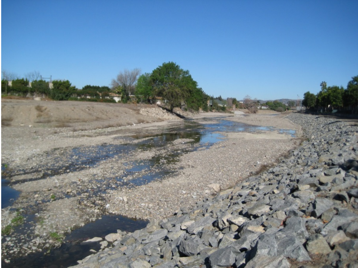
Figure 14-4: Santiago Creek, view upstream from Tustin Avenue in Orange
