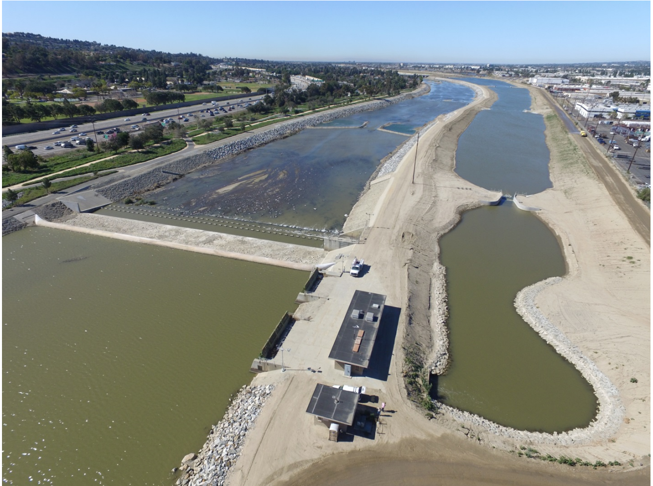
Figure 14-1: View of Santa Ana River (left) with OCWD recharge facilities (right). An inflatable rubber dam that crosses the river here enables OCWD to divert some river flows into basins for percolation.
