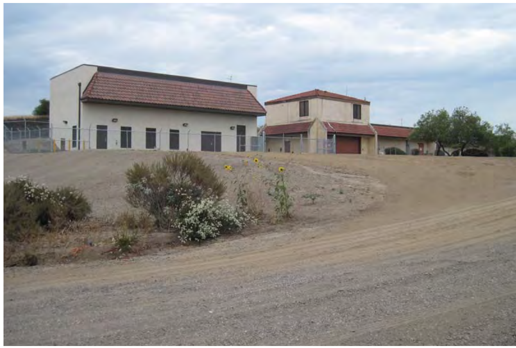
View of non-urban industrial area at the Baker Raw Water Pumping Station.
