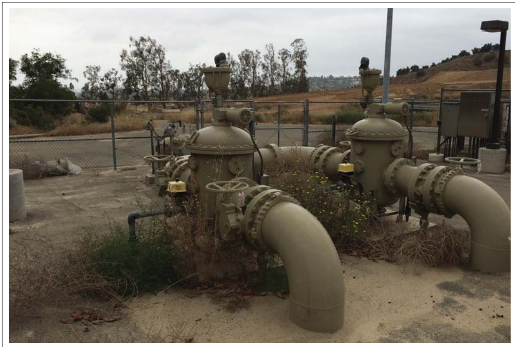
View 1: View of Orchard Hills Facility looking southwest.
