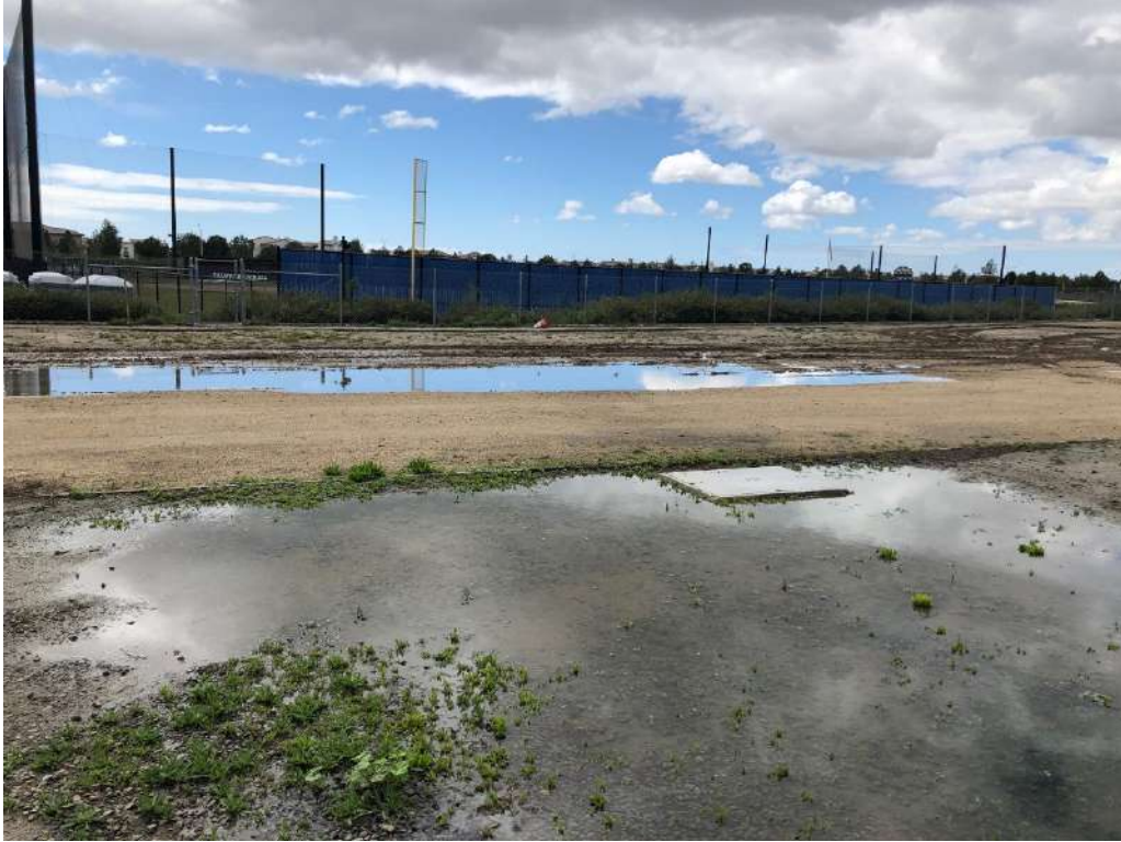
Photo 5: View of puddles near athletic fields (facing south).
