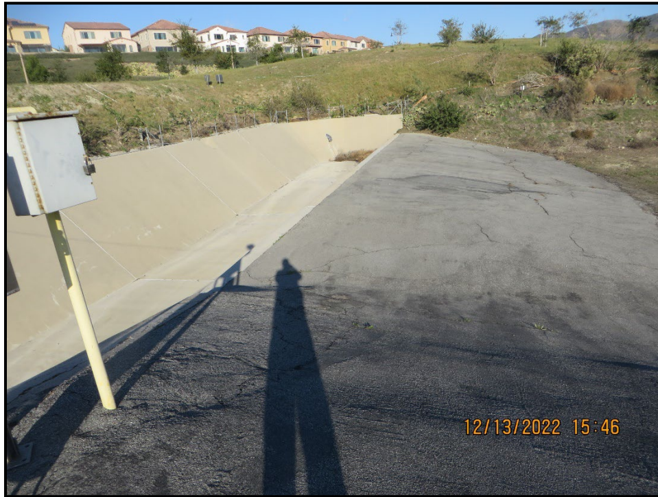
Photo 5) Spillway control section and channel upstream.
