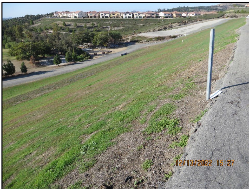
Photo 4) Downstream face looking towards right abutment, photo taken from crest.
