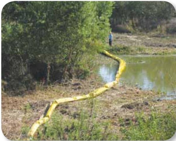
A worker installs the trash boom in San Diego Creek.
