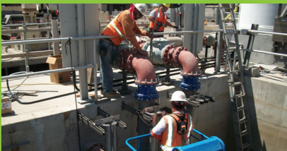
Workers installing the spent backwash tank-pump discharge pipes.
