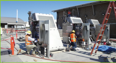
Installation of electrical wiring for the new headworks mechanical screen.
