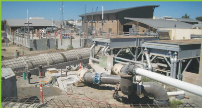
New storm water pump station piping during installation.
