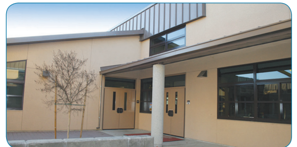
The music and fitness building at Woodbridge High in Irvine Unified School District uses recycled water.
