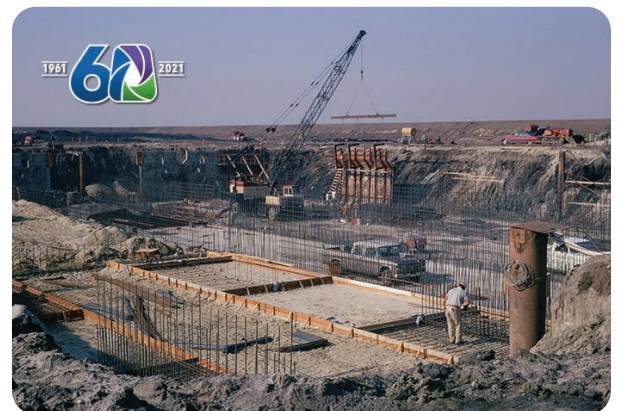
Construction of IRWD's Michelson Water Recycling Plant in the 1960s.
