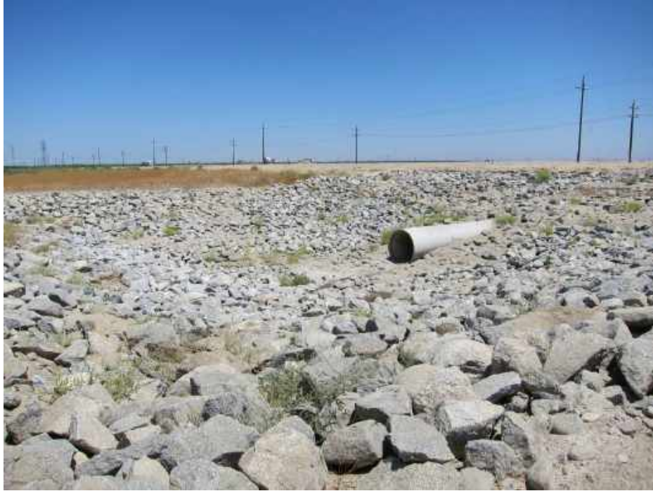
Photo 7 – Photo depicts the culverts associated with the water recharge basins on the Stockdale West property
