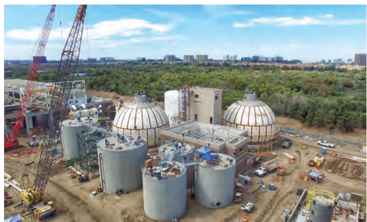
Biosolids and Energy Recovery Facilities Project
