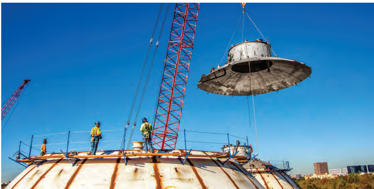
Biosolids and Energy Recovery Facilities Project
