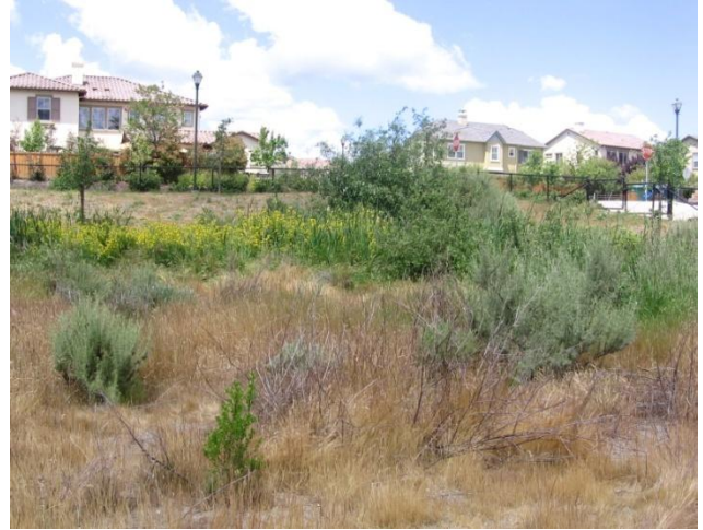
Oval shaped bioretention facility
