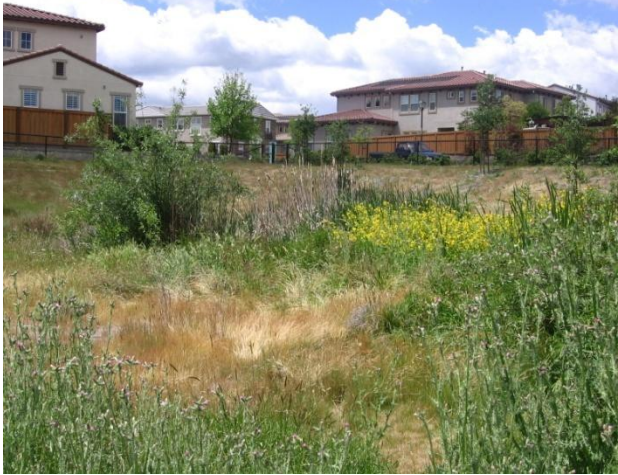
Rectangular shaped bioretention facility
