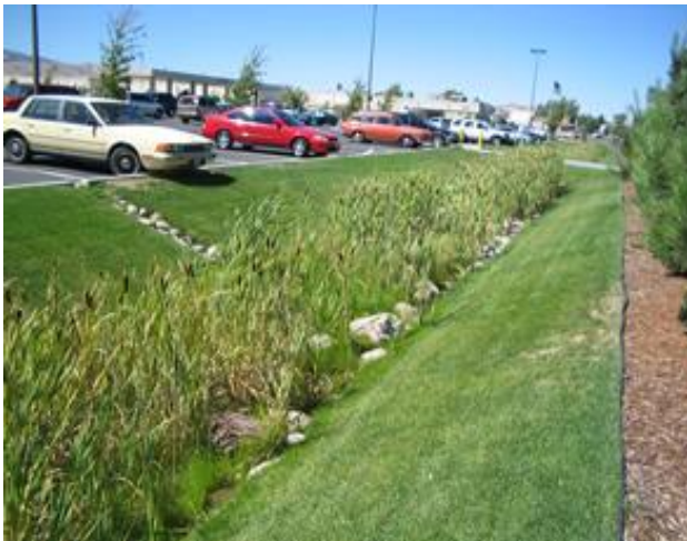
Linear bioretention facility
