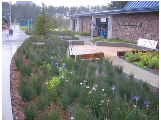
Irregular shaped bioretention facility
