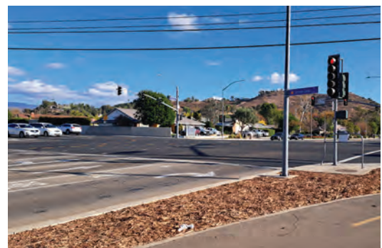
Santiago Canyon Road and Cannon Street will present existing utility crossing and traffic control challenges.
