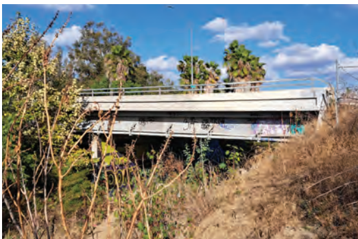
The County of Orange will require an encroachment permit for the pipeline to cross Santiago Creek.
