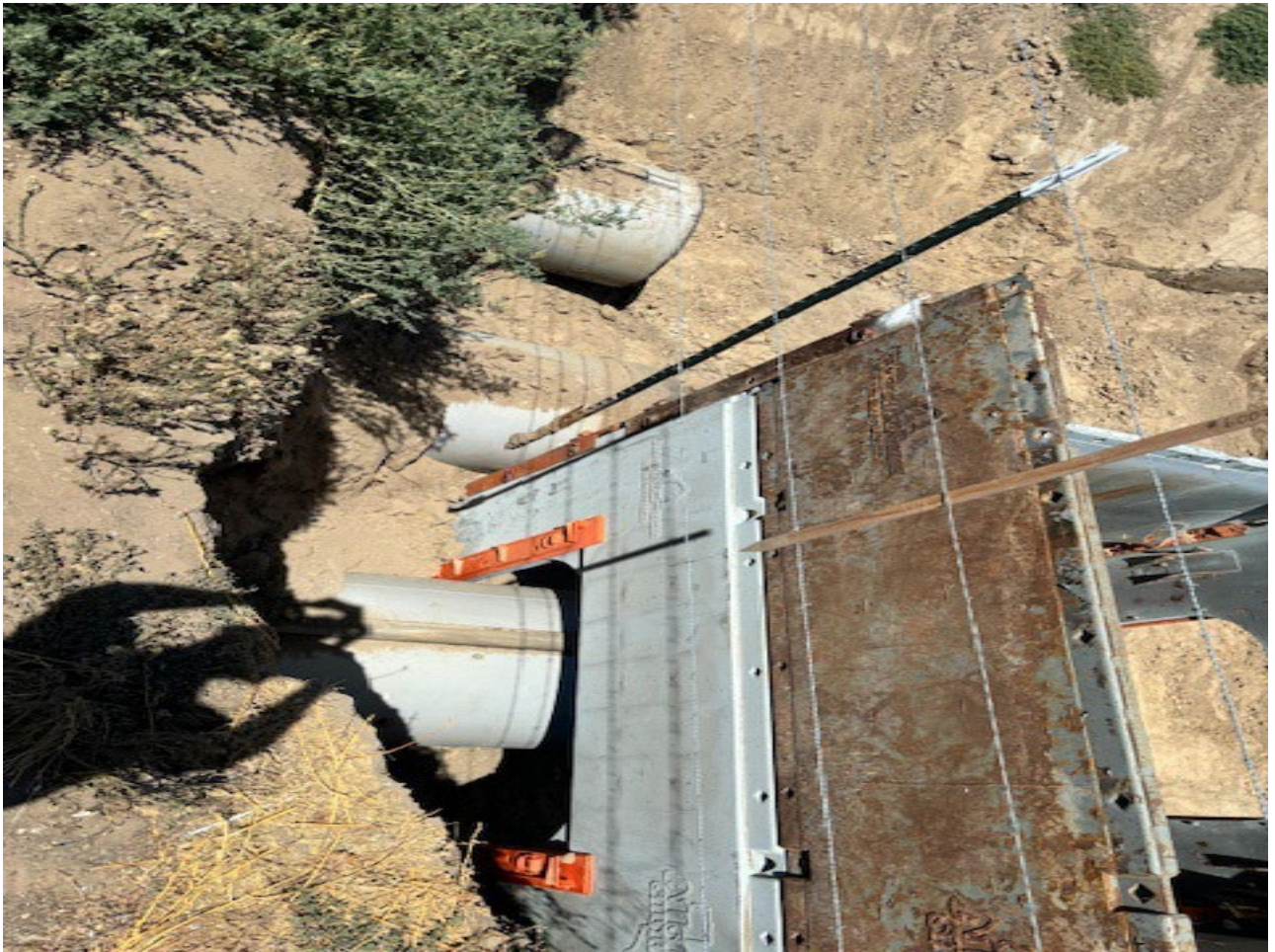
Casing Receiving Pit Entrance
