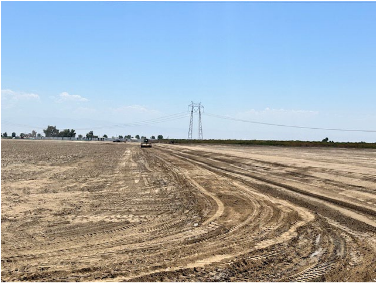
Levee Embankment Fine Grading
