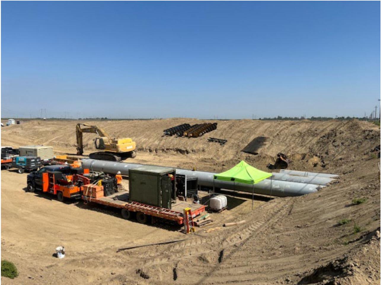
Casing Pipe #3 Installation
