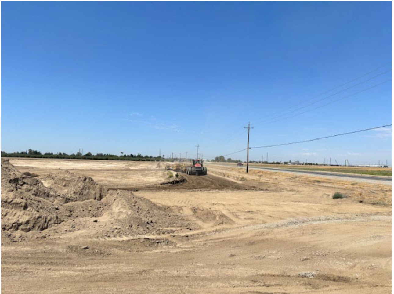
Levee Over-Excavation and Recompaction
