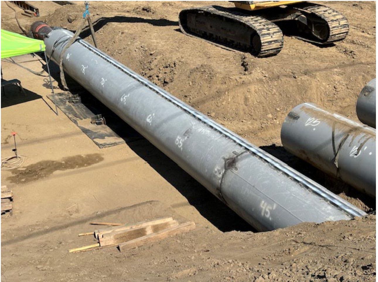
Casing #4 Installation
