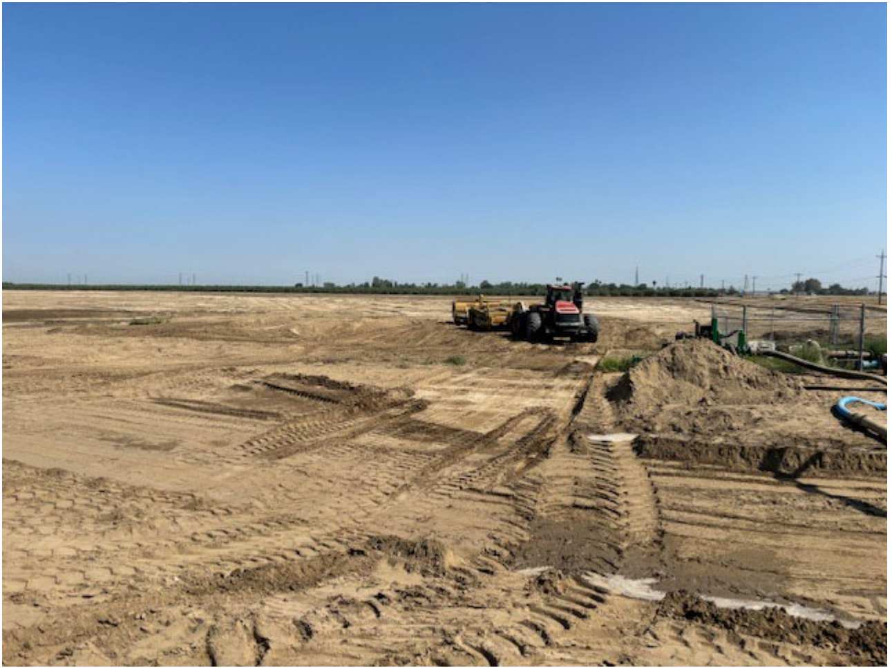
Subgrade Preparation for Levee Embankment around Existing Well
