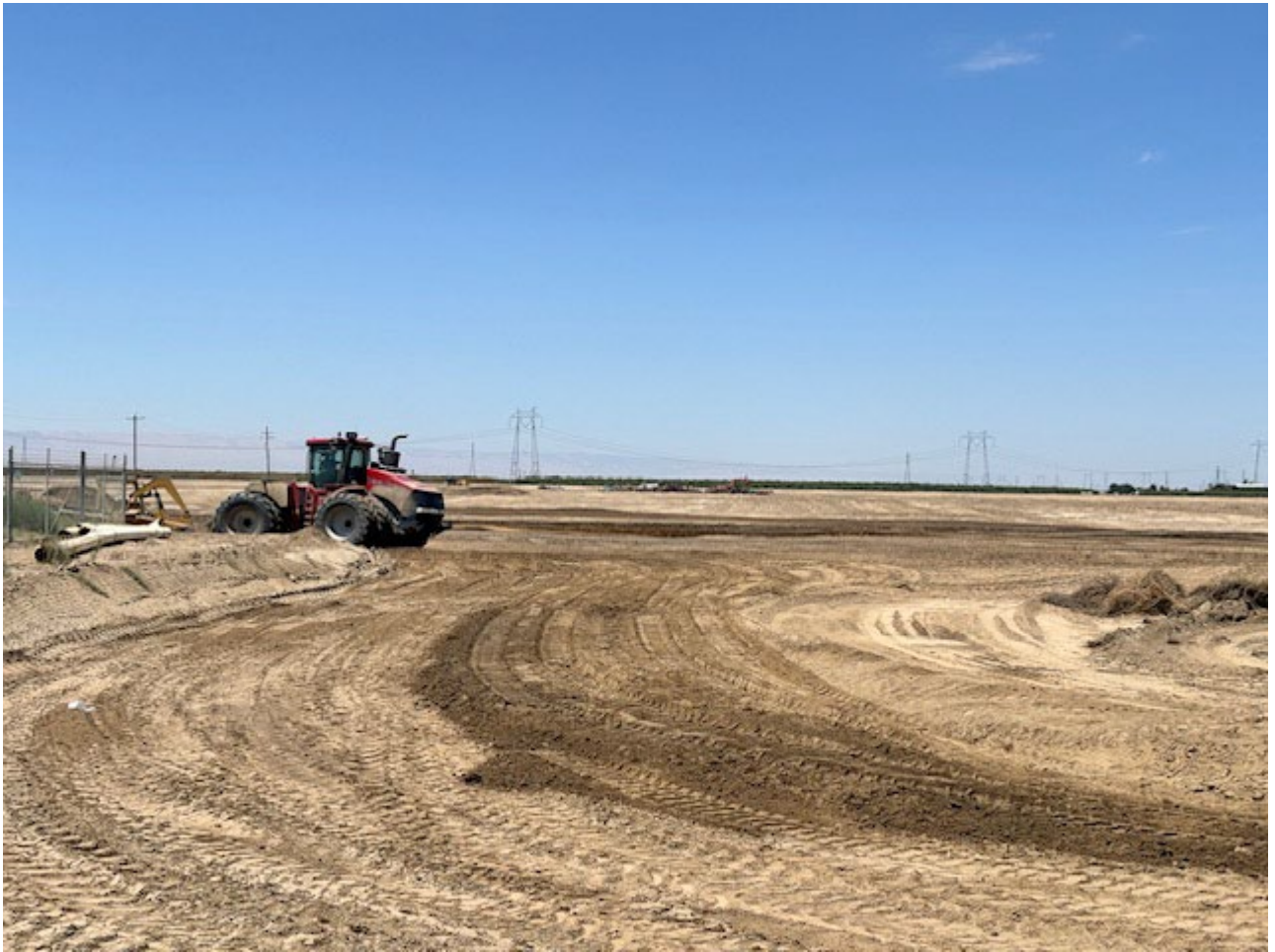
Backfill and Compaction of Levee Embankment Keyway around Existing Well
