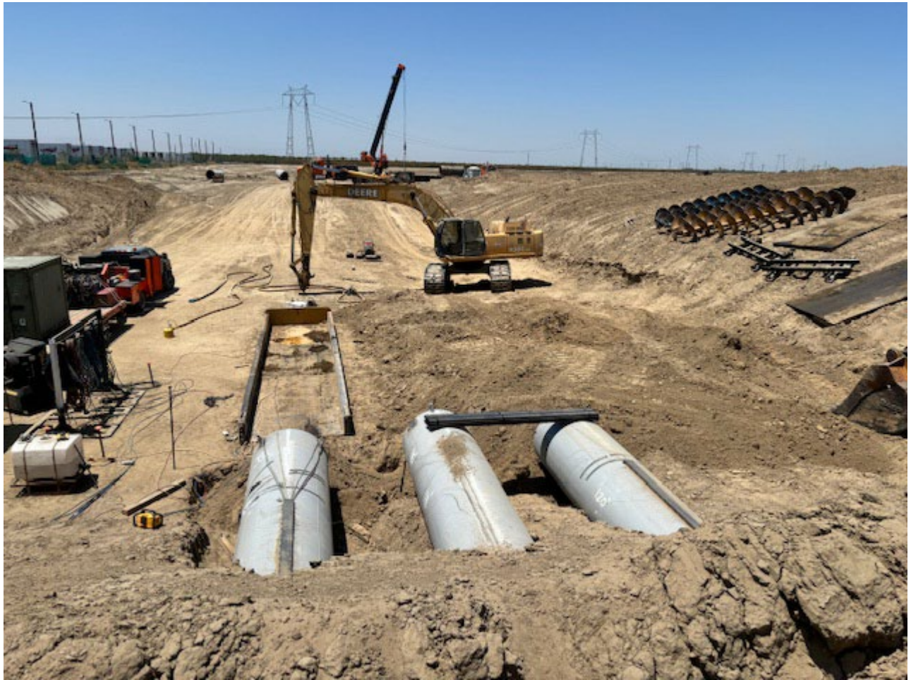
Completion of Third Casing
