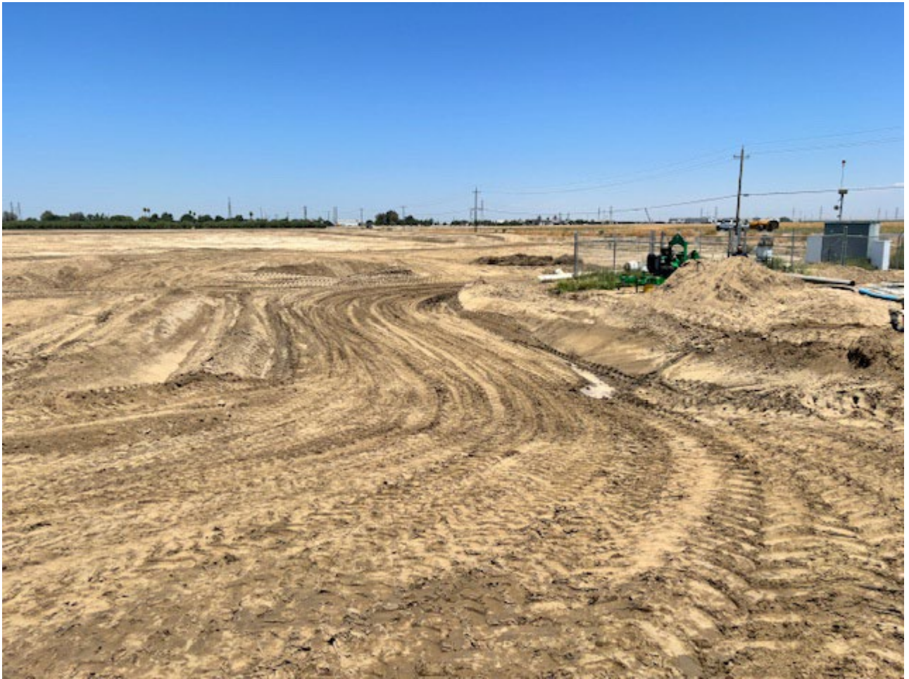
Levee Over-Excavation and Recompaction
