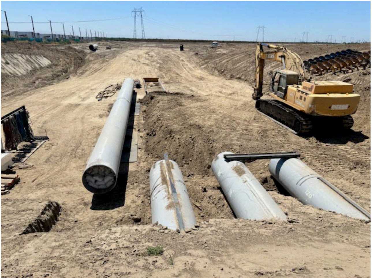
Preparation for Installation of Cased Crossing #4
