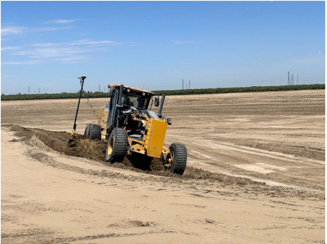
Fine Grading Levee Embankment Slopes
