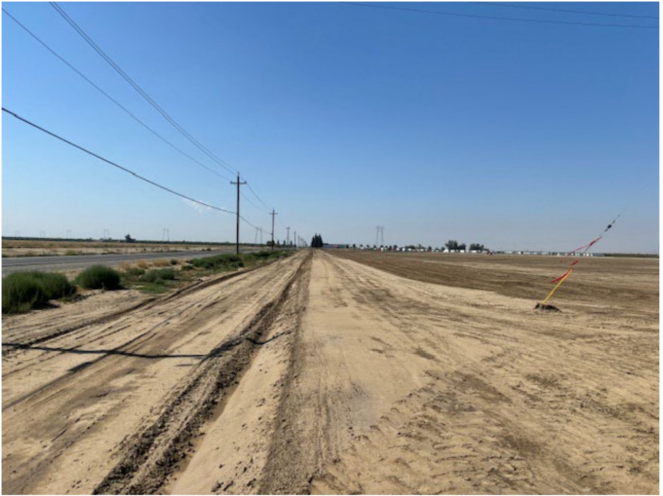
Levee Embankment Fine Grading
