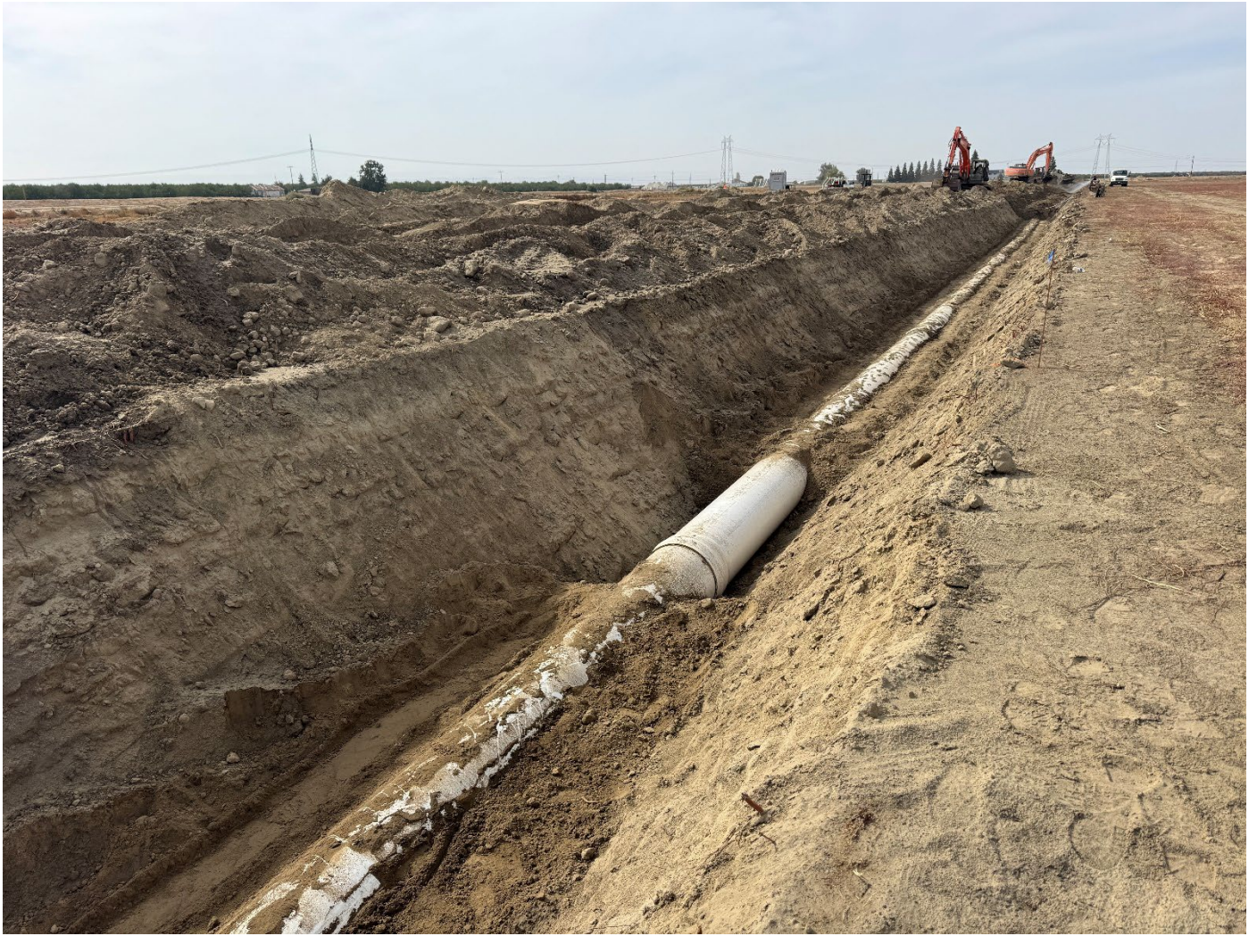
Compaction Efforts Around Pipe Zone, Location of Air Release Valve
