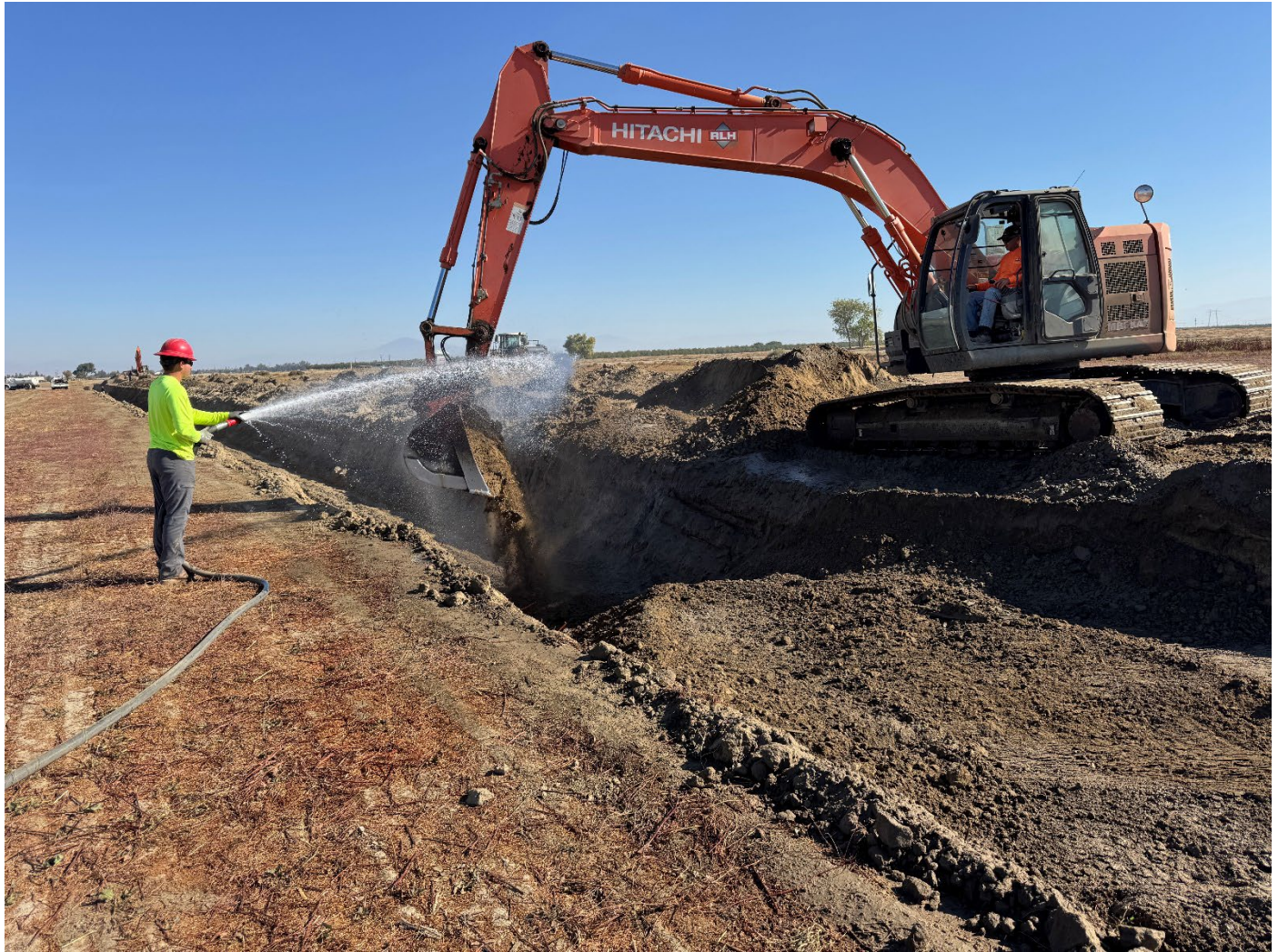
Backfilling above pipe around STA 75+00
