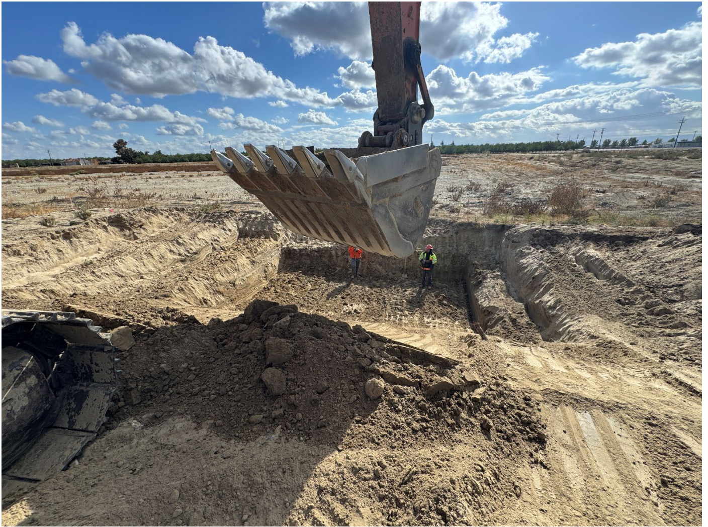
Excavating Basin Structure Bottom for Goose Lake Turnout
