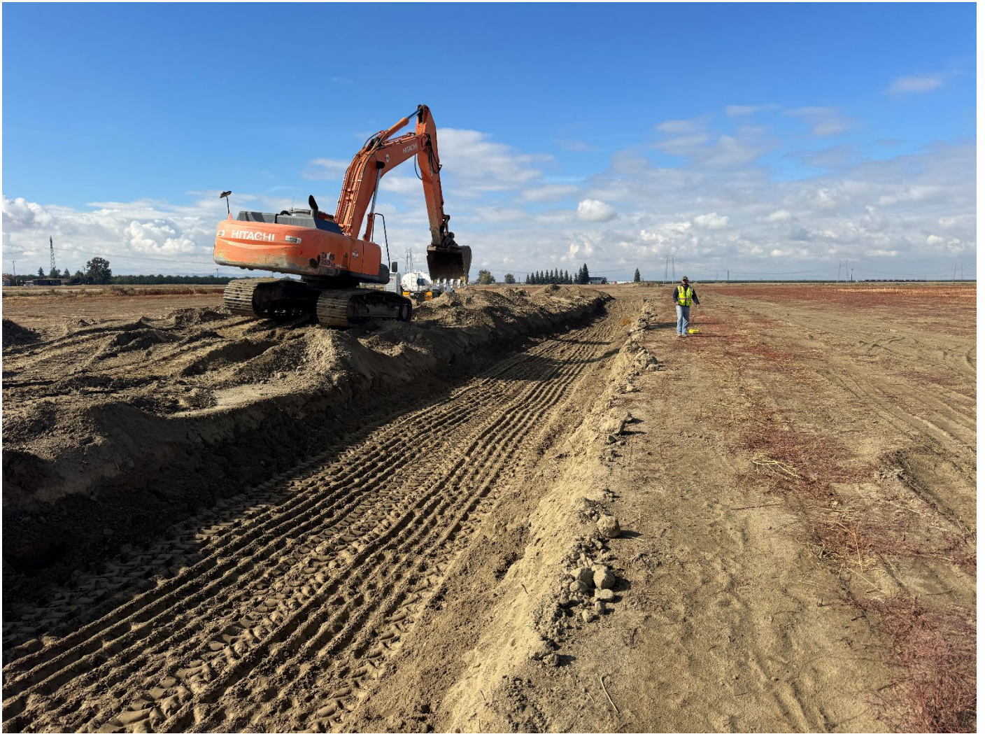
Trench Backfilled Two Feet Above the Pipe
