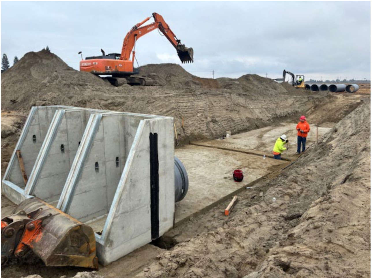
Goose Lake Turnout Structure
