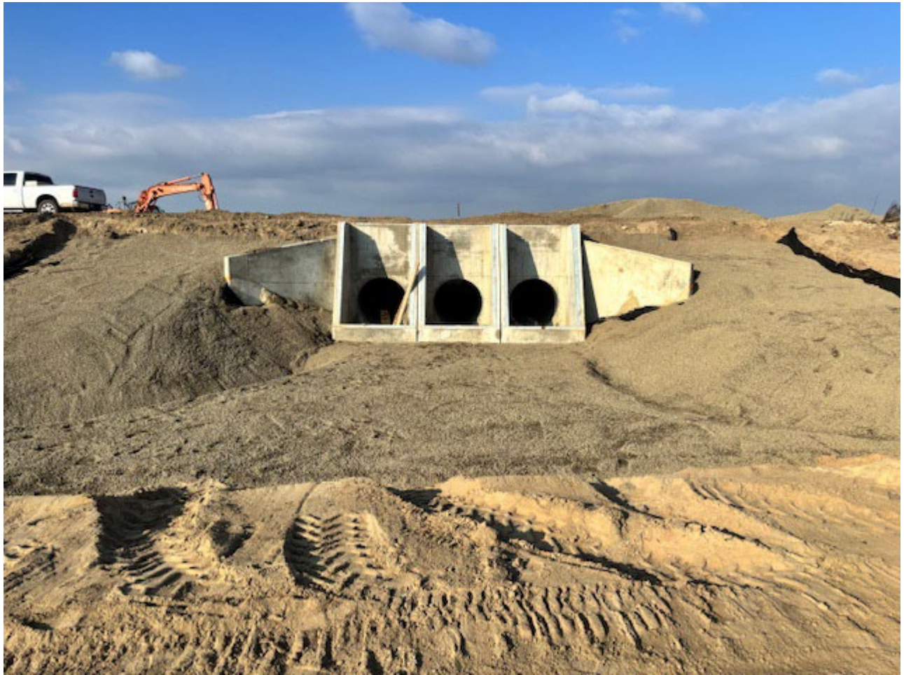
Gravel Rock and Fabric Upstream of Goose Lake Turnout Structure
