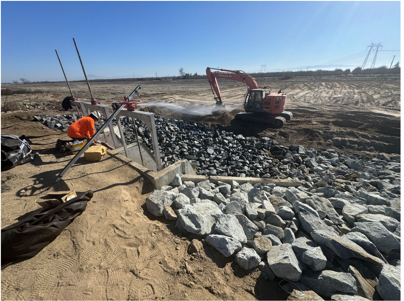
Rip-Rap Installed at Inlet Channel of Goose Lake Slough Turnout
