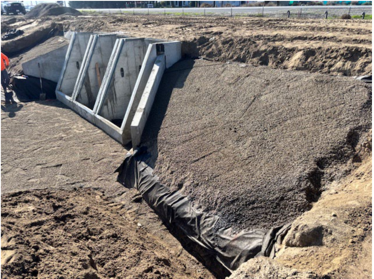
Placing Fabric and Gravel Rock at West Enos Turnout Structure
