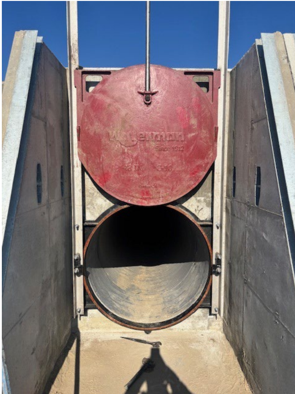
Slide Gate Installation
