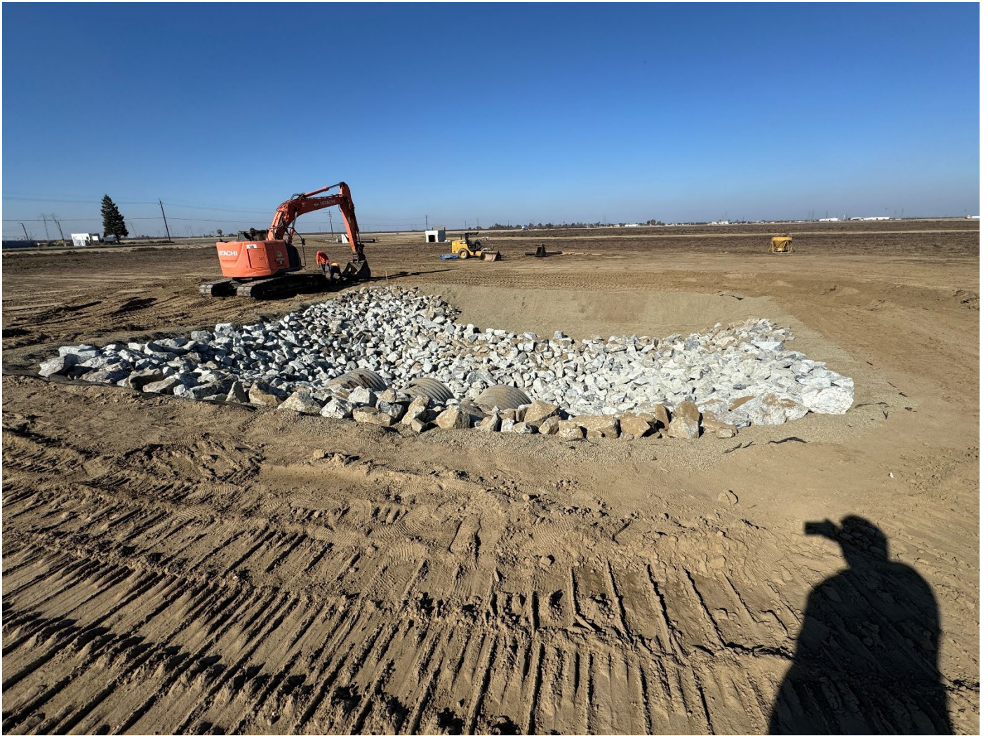
Rip-Rap Installation at Outlet Channel of Goose Lake Slough Turnout
