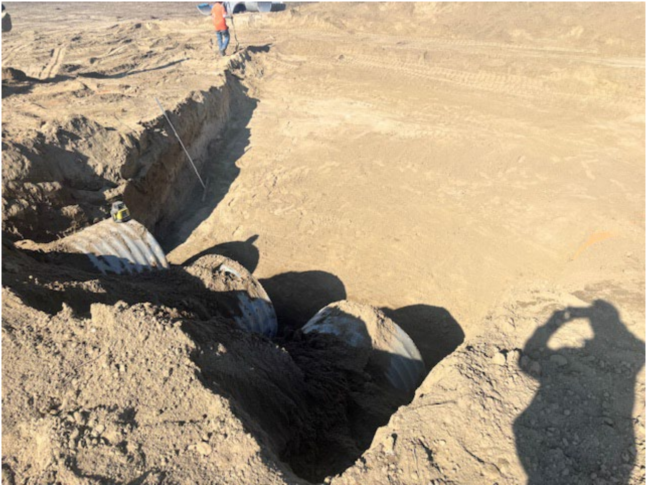
Excavation for Outlet Channel from Goose Lake Turnout
