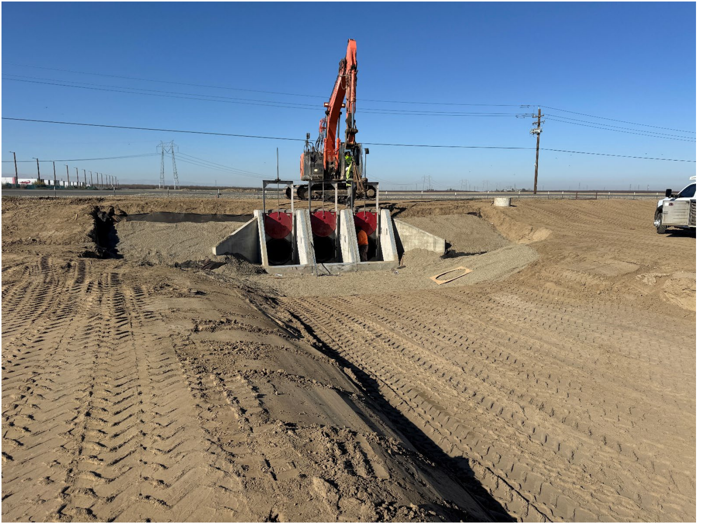
Finishing Installation of Slide Gates
