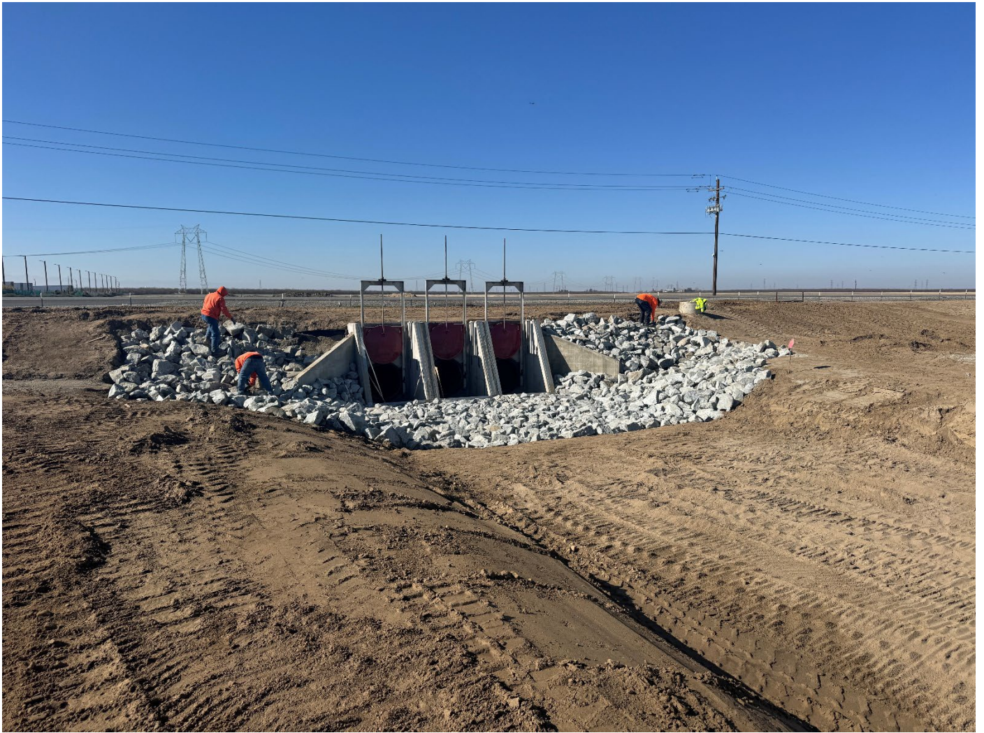
Rip-Rap Placement at West Enos Turnout
