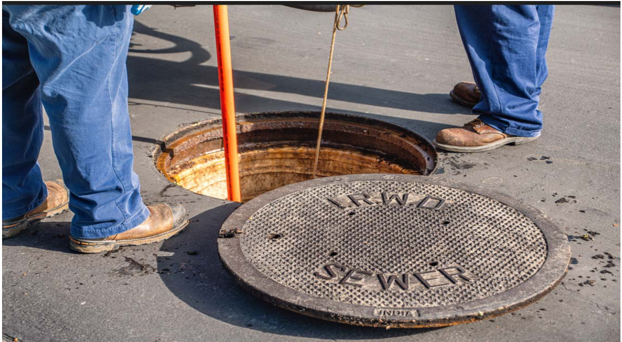
IRWD Manhole Cover
