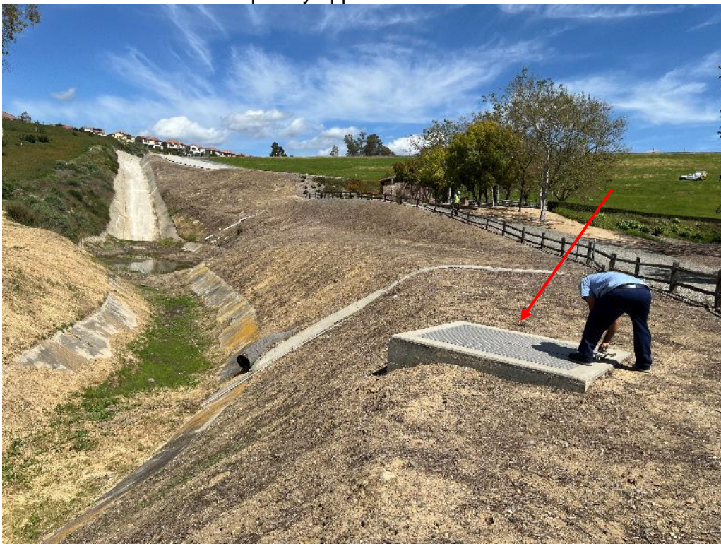
Photo 4. Location of drain outfalls 2, 3, 4, 5, 8, and 11.
