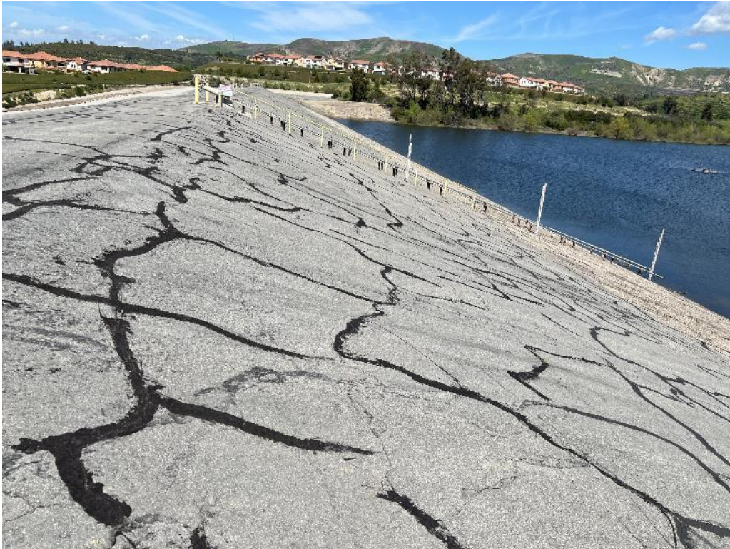
Photo 2. Upstream face of the dam.
