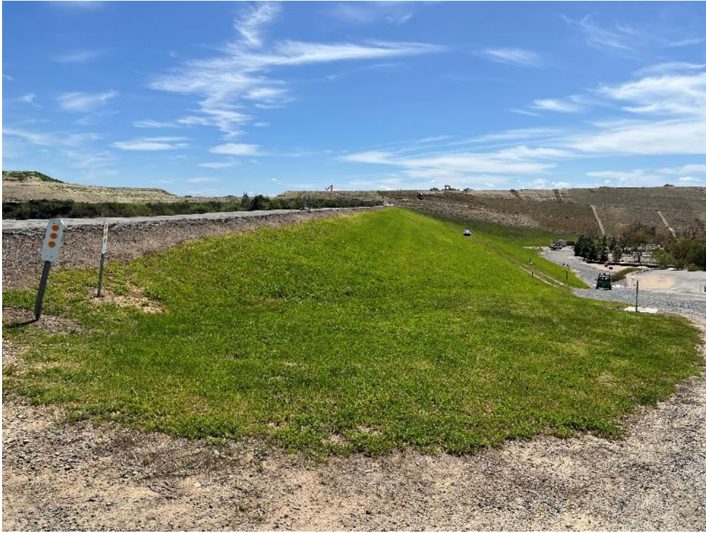
Photo 1. Downstream face of the dam.
