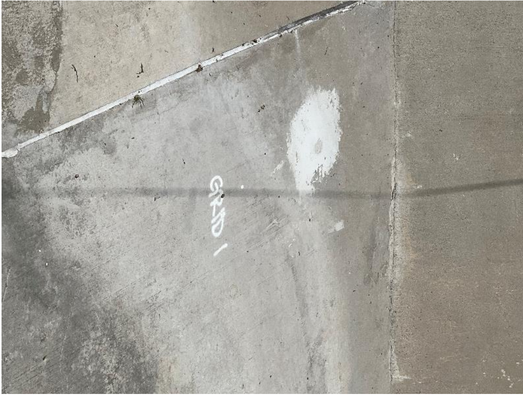
Photo 7. Example of backfilled boring in the spillway.
