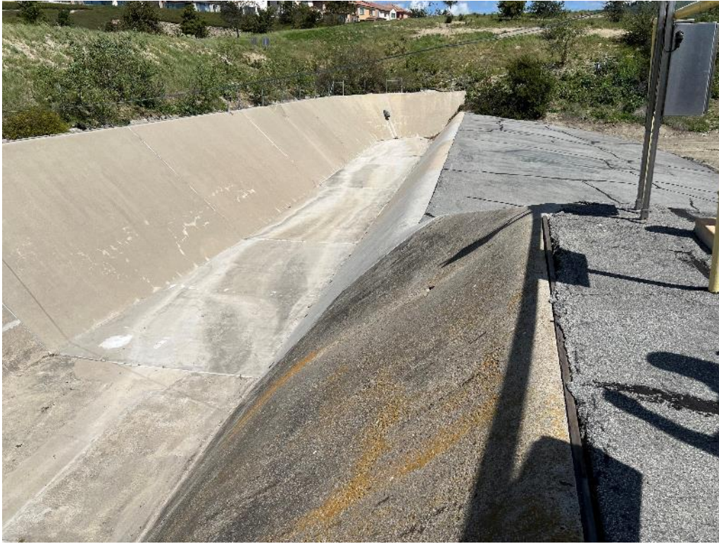
Photo 3. Spillway approach and side channel.
