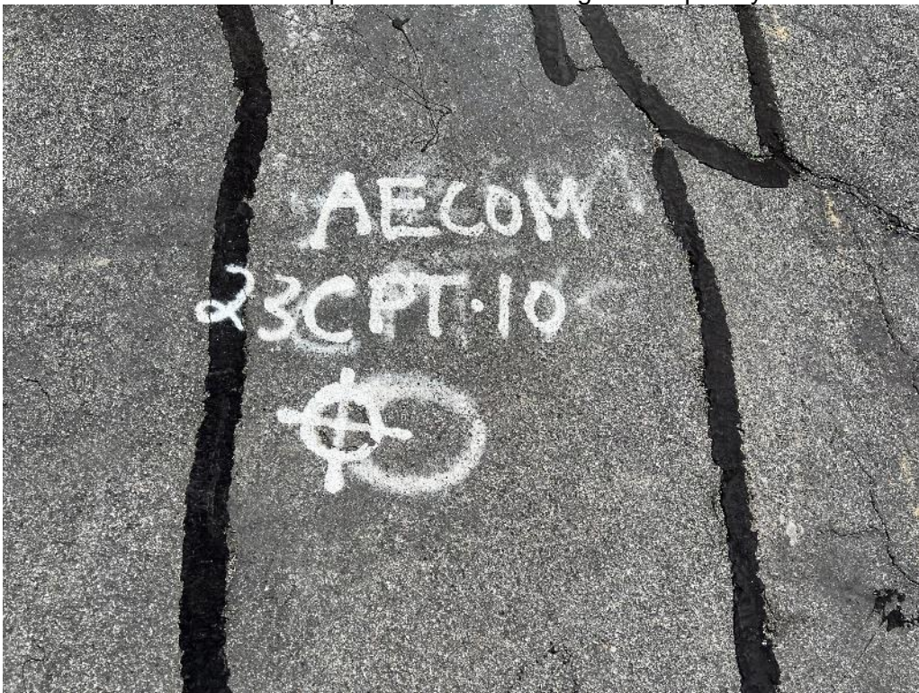
Photo 8. Example of backfilled boring in the crest.
