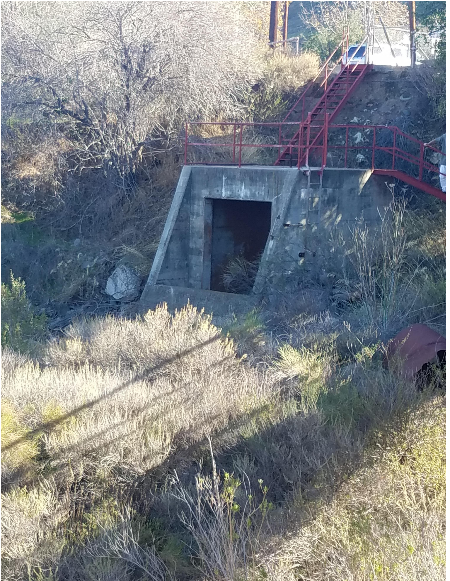
Exhibit 6.5 Location of Critical Valve at Santiago Creek Dam
