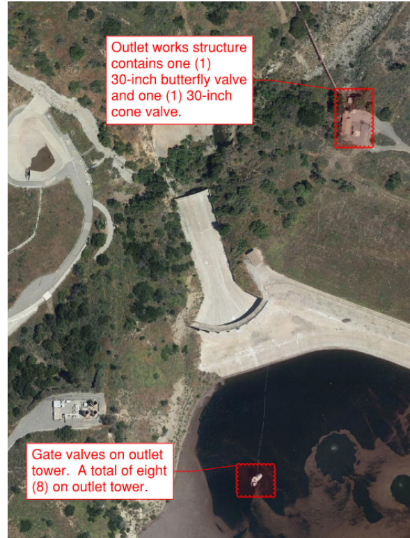
Figure 1: Santiago Reservoir valve locations for releasing water to Santiago Creek.
